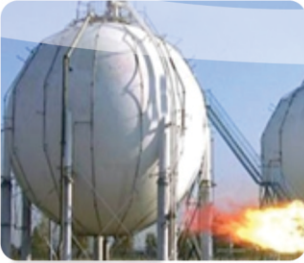
Jet fire protection
